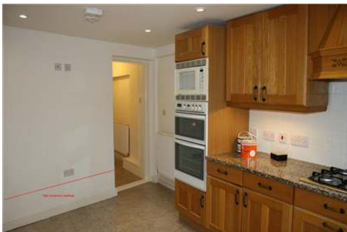
Kitchen - damp in original external wall
