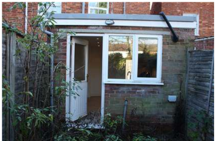
Rear wall - brickwork looks damp
