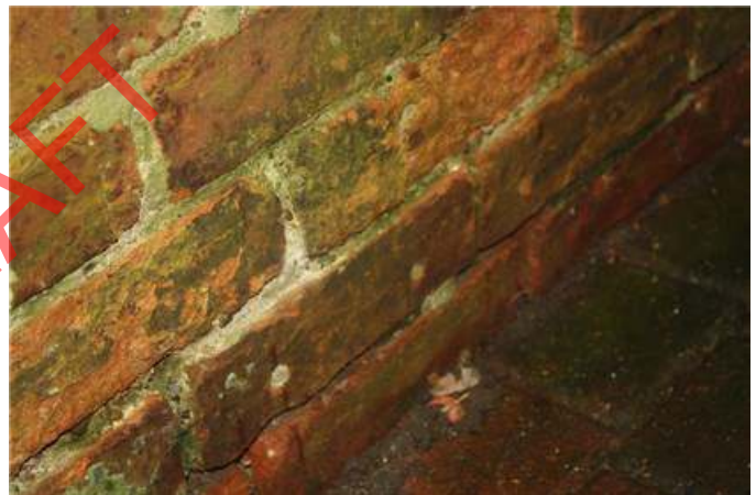
Side elevation wall - injected dpc
