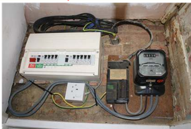
Electric meter and consumer unit
