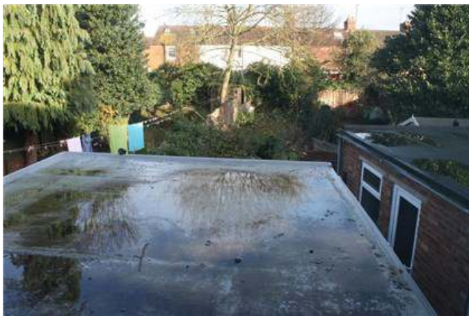
Flat roof to kitchen - rainwater is pooling
