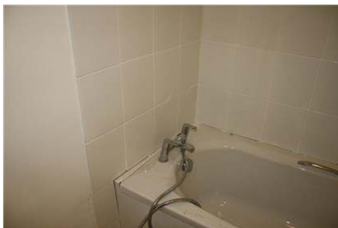
Sealant missing around bath
