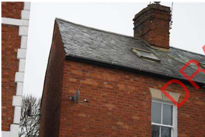
Gable wall - leaning out slightly at top
