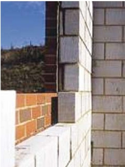
Fig1—Modern brick/block cavity wall
