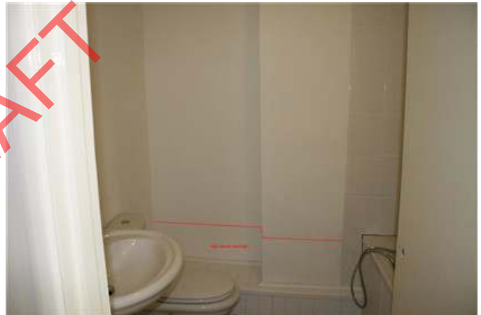
Bathroom - damp in the party wall and chimney breast
