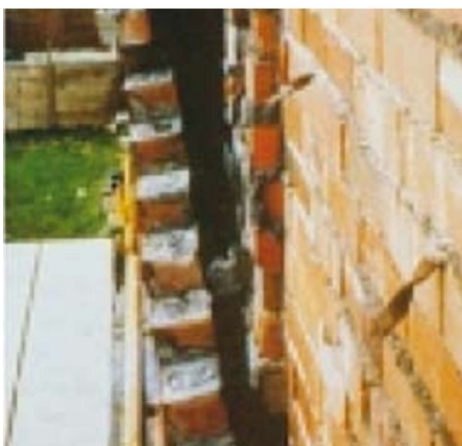
Fig5—Separation of outer leaf
