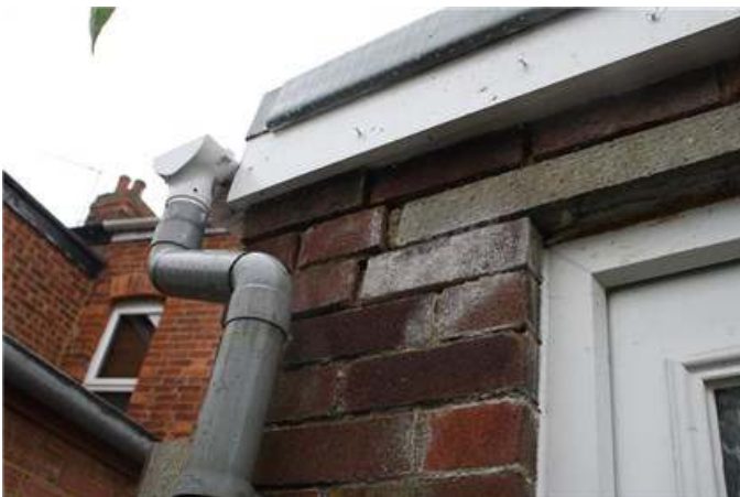
Kitchen rear wall - mortar missing
