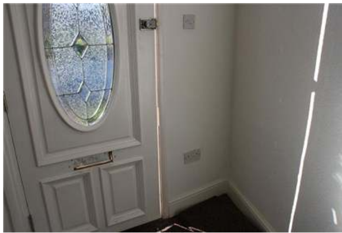
Front door will not close without force
