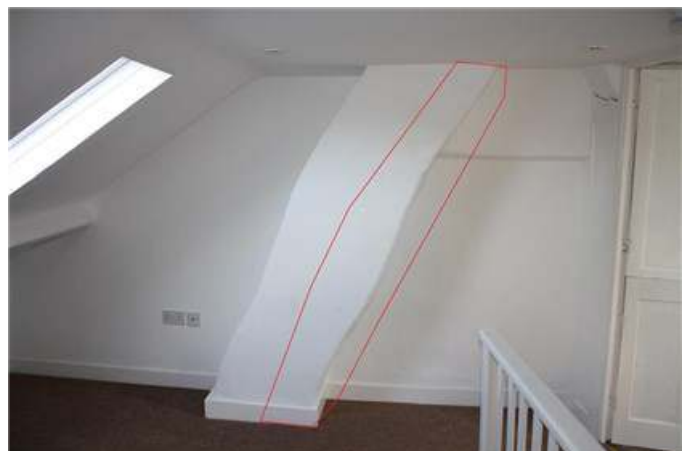
Rear 2nd floor bedroom - damp in chimney breast
