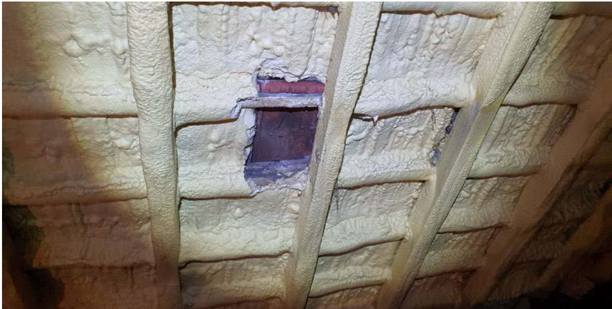
Figure 1: Spray foam used to stabilise a failing roof cover; a thin coating with limited heat retention but significant water problems
